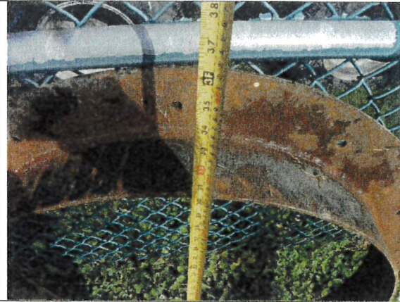
New exterior roof vent 30" flange.
