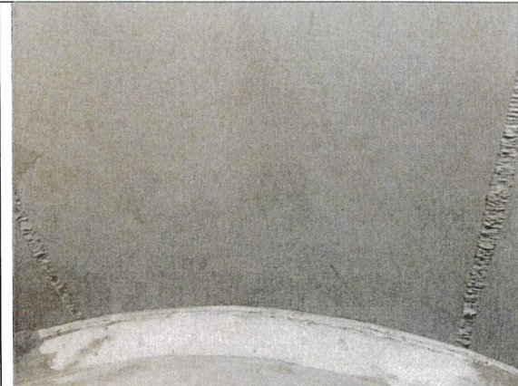
Blast cleaned wet interior dome bowl troth.
