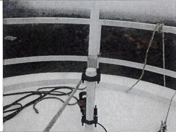
Exterior pressure washing roof.
