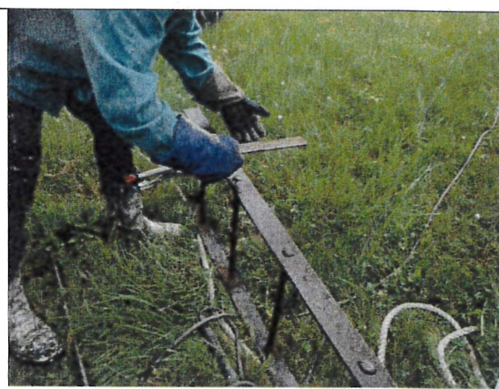
Wet interior ladder assembly started.
