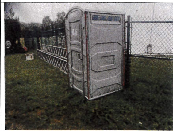
Porta-john brought to site.
