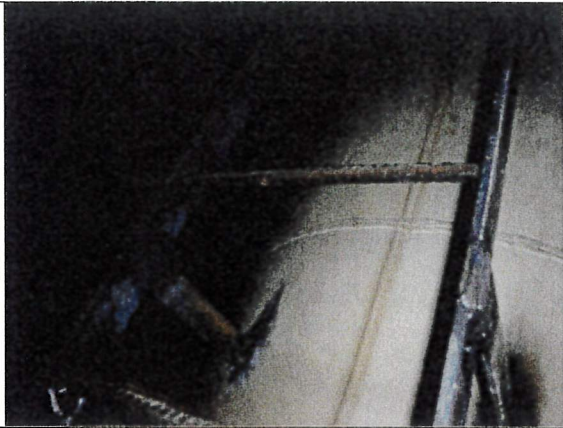
Wet interior ladder welded in place.
