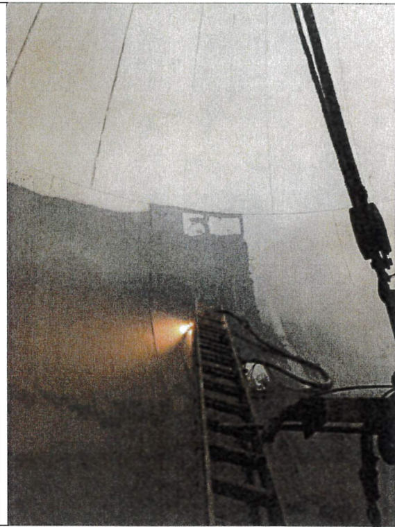
Interior wet blast up to equator on half of tank.
