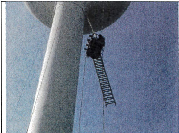
Taking up boom ladders.
