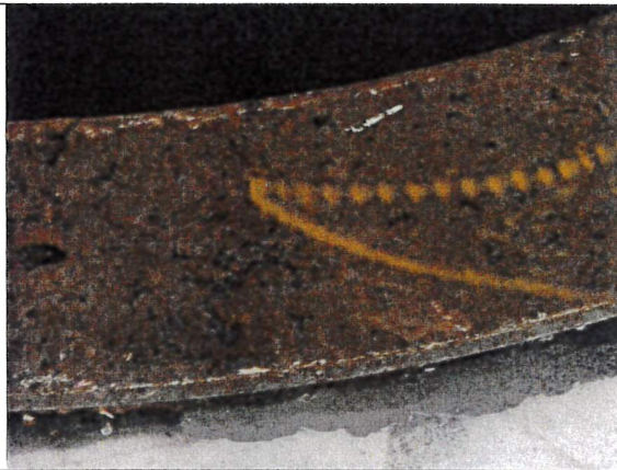
Exterior roof vent flange welded in place.
