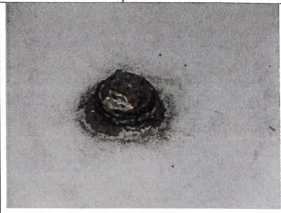
Roof couplings welded in place.
