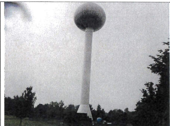
Exterior view of the Waynesville tank.
