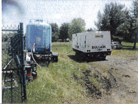
Compressor and blast pot readied.
