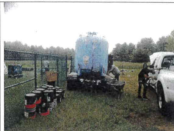
Blast pot on site.
