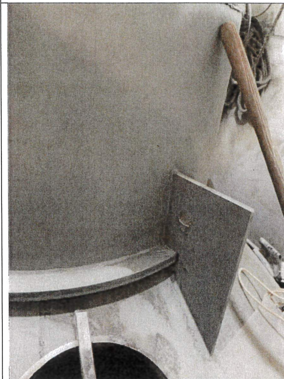
Blast cleaned wet interior dome and riser.
