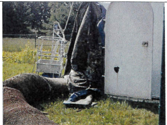
Dust collector put in place.
