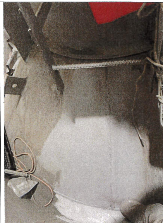
Blast cleaned wet interior dome and bottom of ladder.
