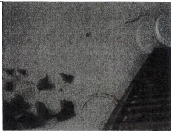
Condition of existing on upper tank.
