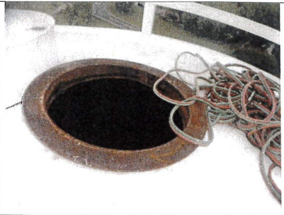
Exterior roof vent flange welded in place.
