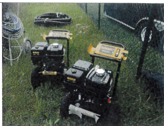
Pressure washing equipment on site.
